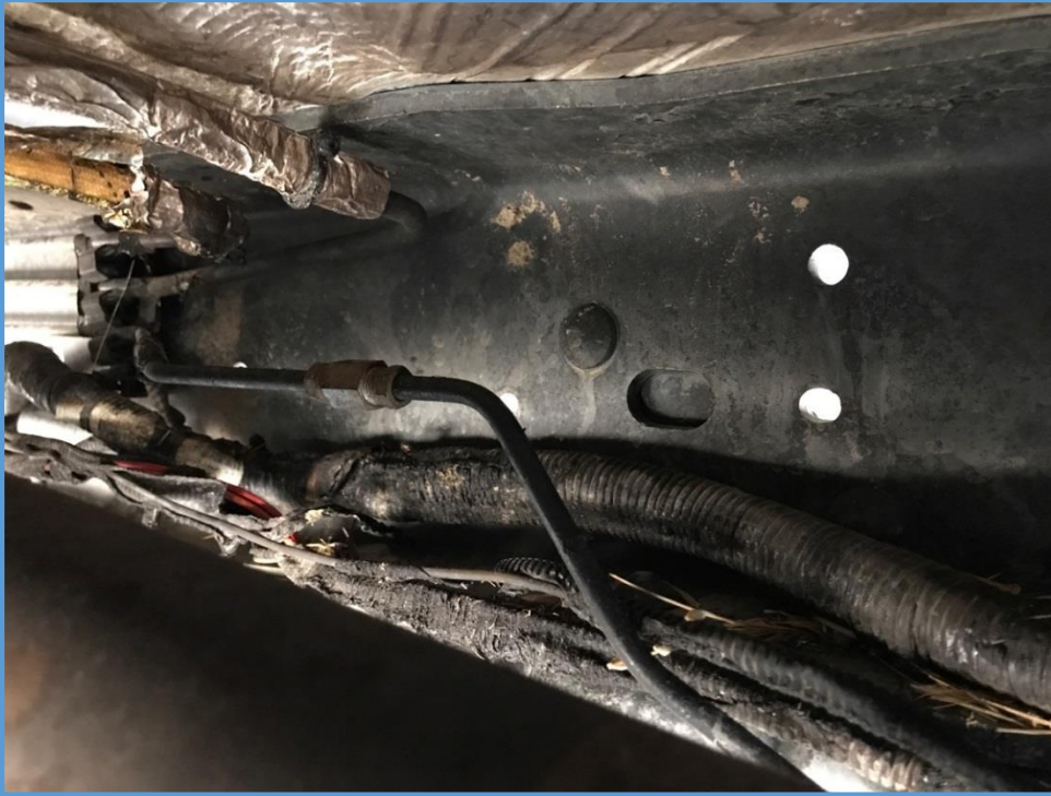
E-521 burn damage occurred to: the wiring harness located on the driver's side of the frame, the wiring above the transfer case, and two plastic/rubber fuel lines.
